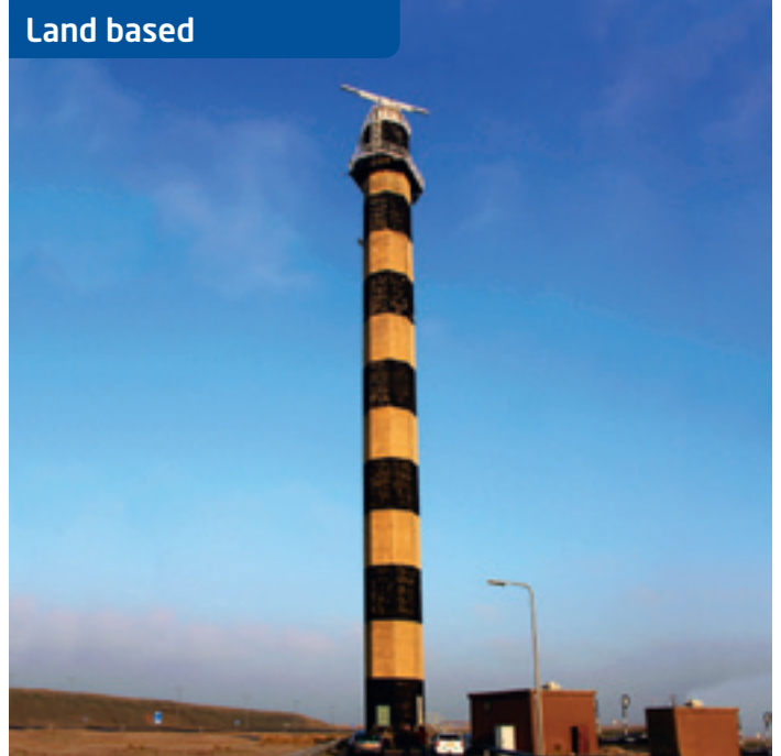
Fixed radars mounted on land can both monitor oil on surface and gather hydrographic information. A tall mounting tower is required to obtain maximum operational range.
